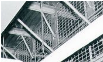
Factory made cutouts fit around building structure.
